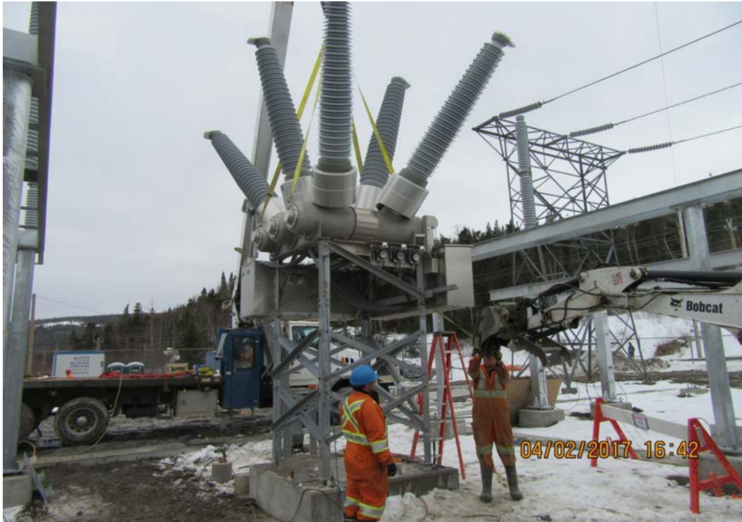
Bay d'Espoir Terminal Station 2 – Circuit Breaker Installation
