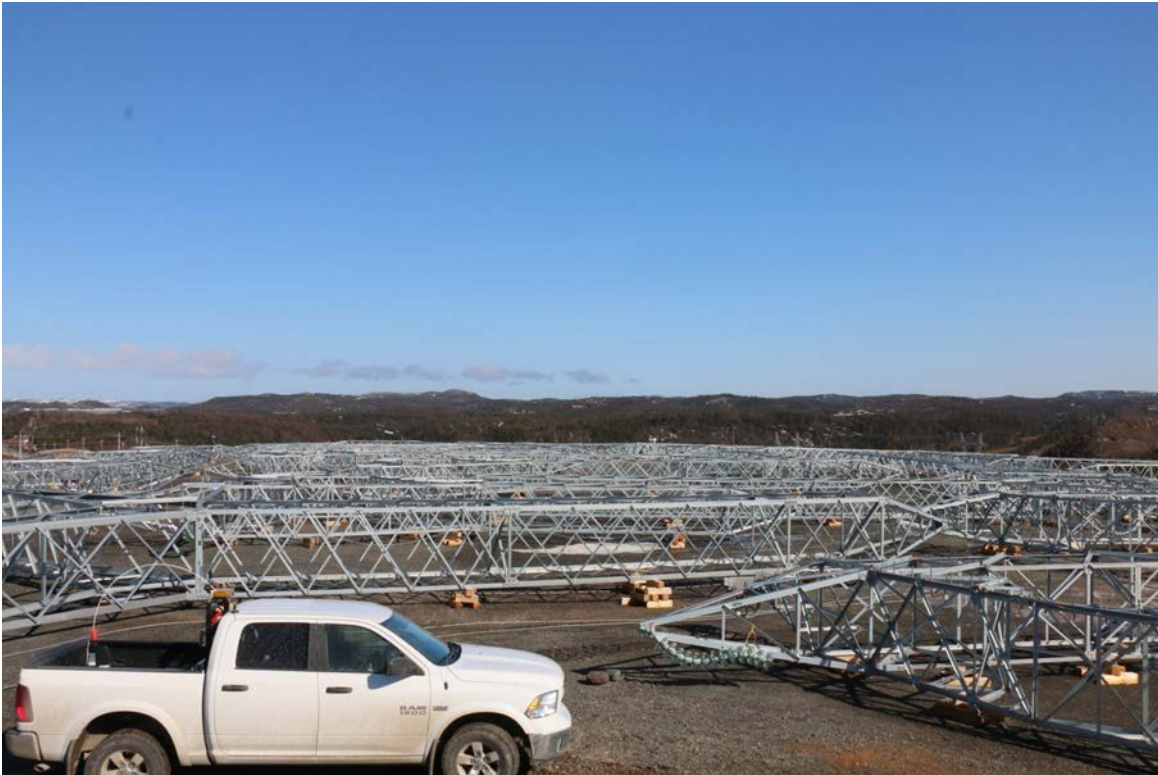
Tangent Tower Assembly Yard (Fly-yard)
