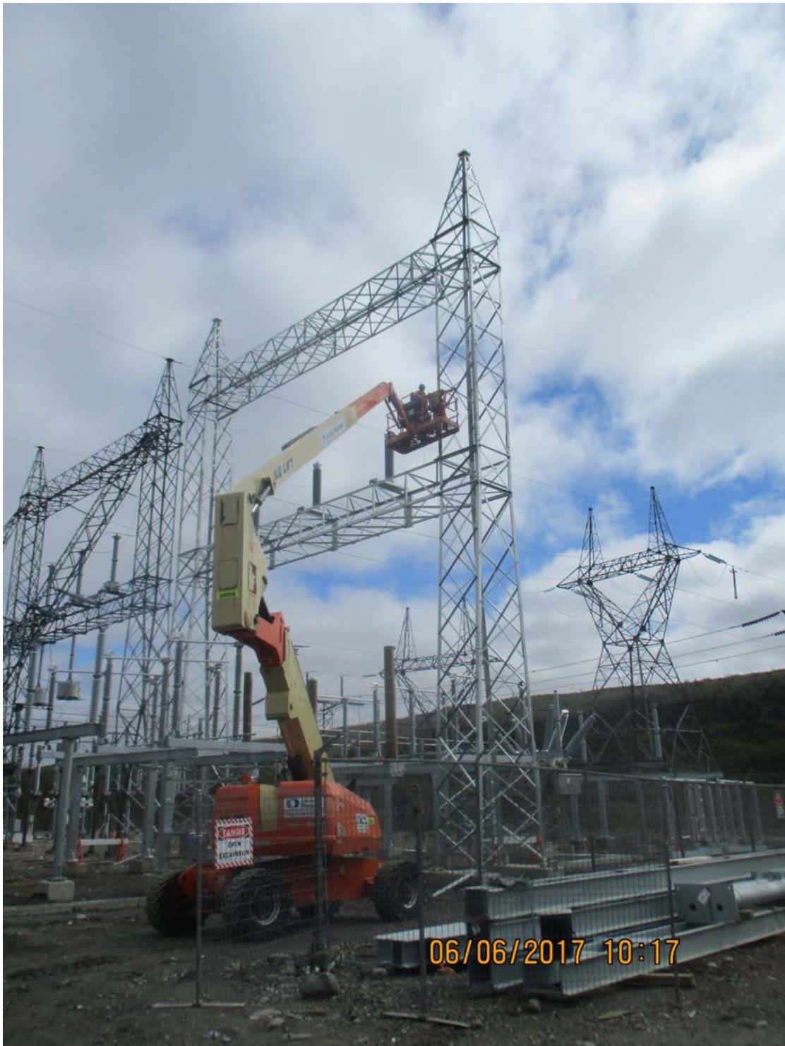
Bay d'Espoir Terminal Station 2 – Gantry Construction
