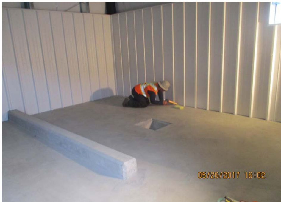
Finishing Building Interior in Bay d'Espoir Terminal Station 2
