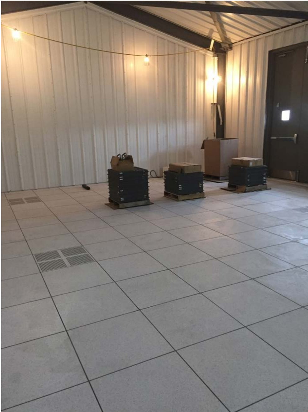
Western Avalon Terminal Station – GIS Building Interior Fit-up
