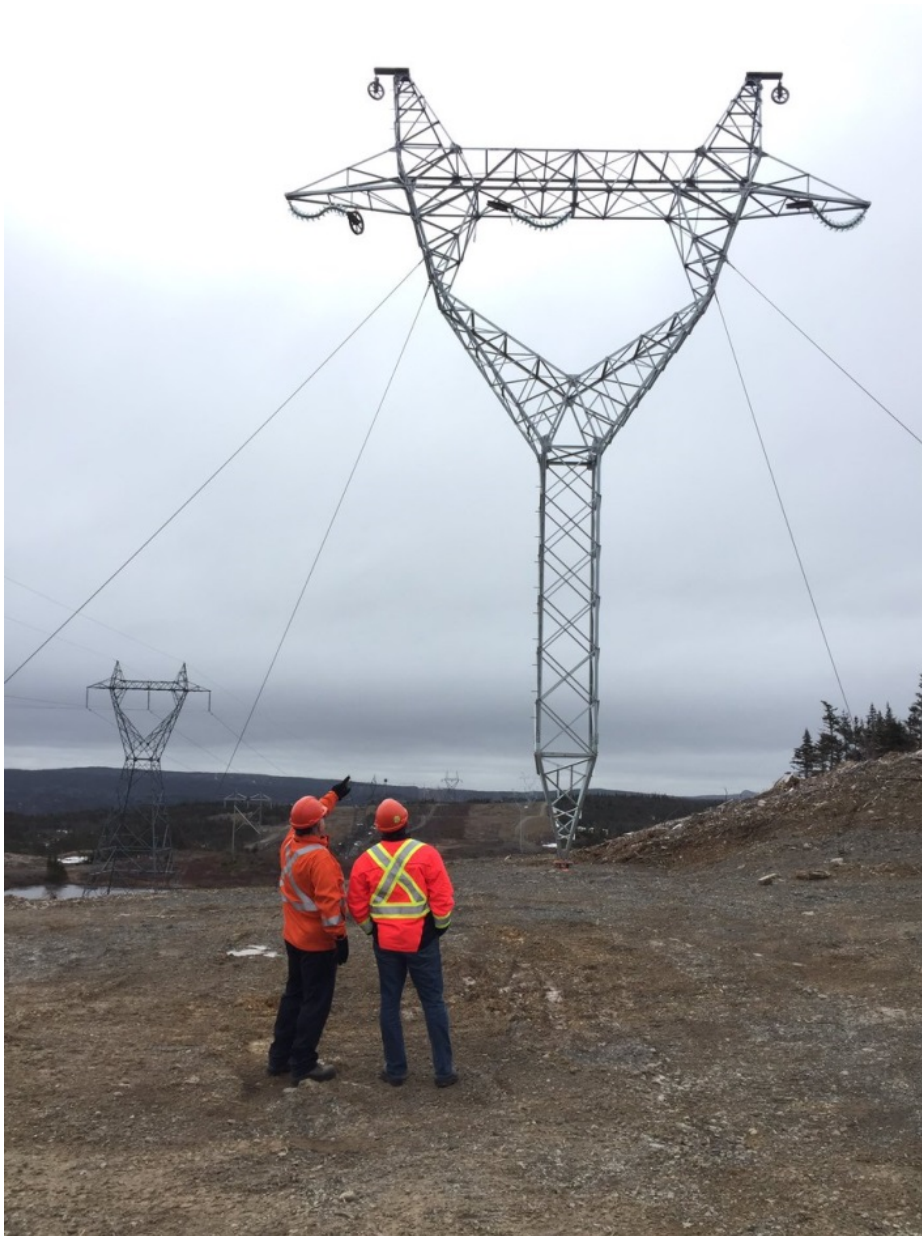
Completed Tangent Tower
