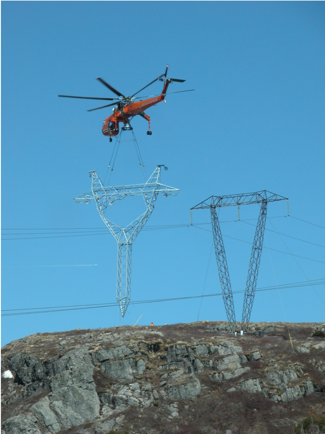
Tangent Tower Erection by Air-Crane
