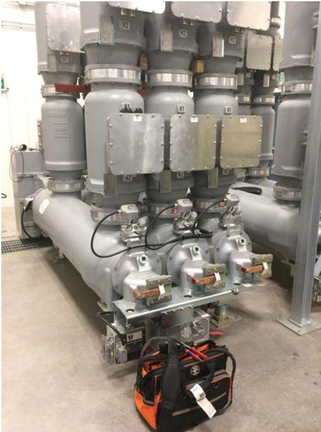
Western Avalon Terminal Station – GIS Equipment Installation
