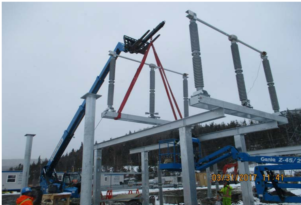
Bay d'Espoir Terminal Station 2 – Disconnect Switch Installation
