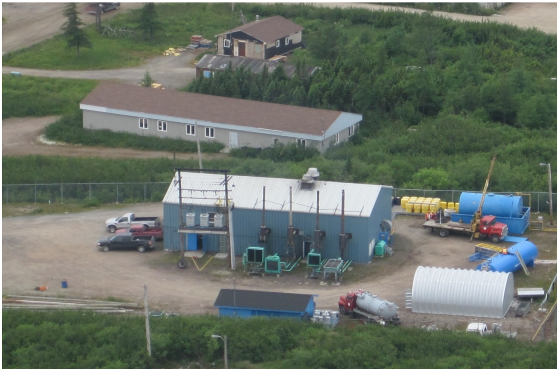
Figure 1: Cartwright Diesel Generating Station
