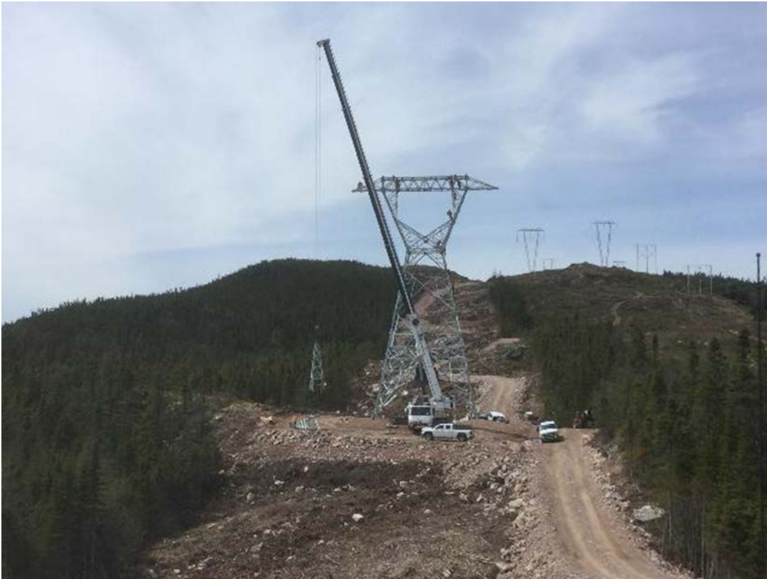
Self-support Tower Erection
