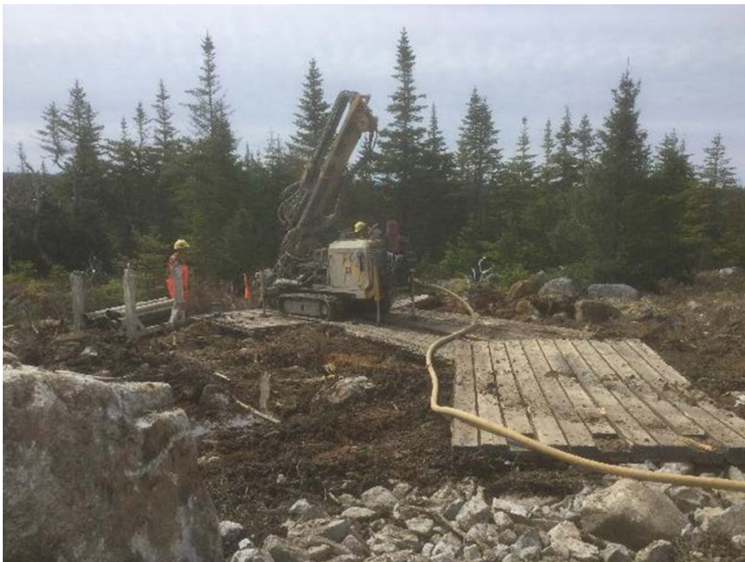
Anchor Drilling Operations
