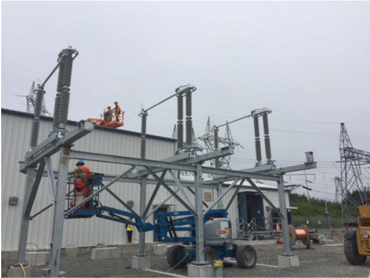
Western Avalon Terminal Station – Disconnect Switch Installation
