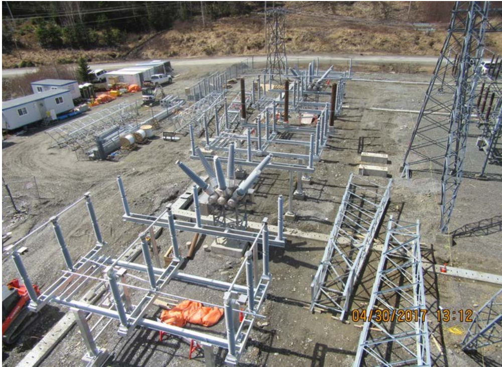
Bay d'Espoir Terminal Station 2 – Equipment Installation
