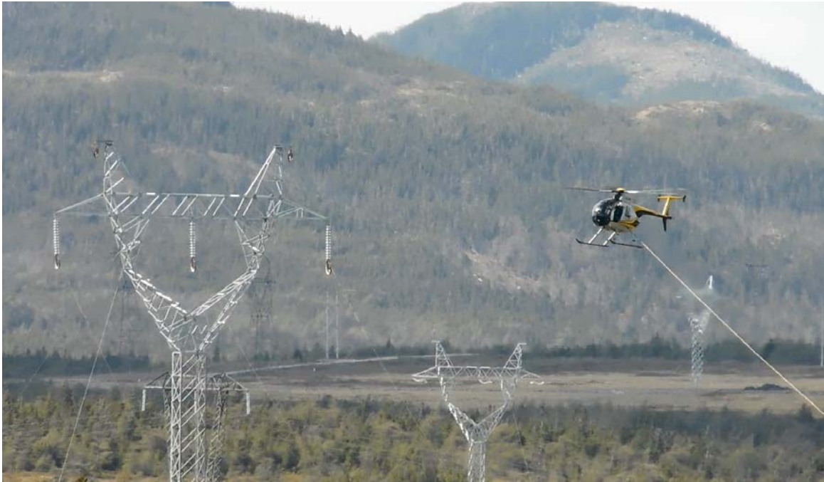
Helicopter Stringing Operations
